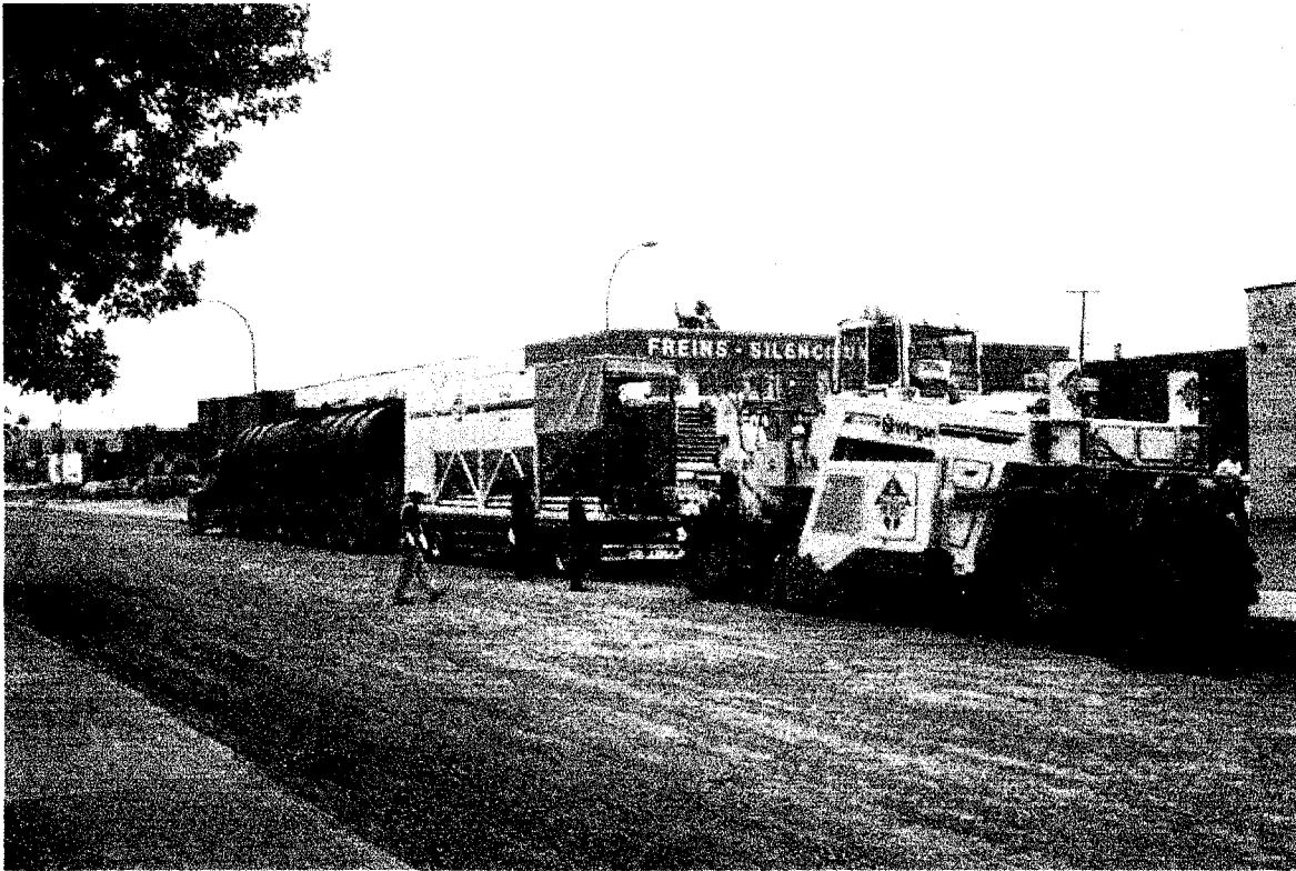
Figure 15 Deep Cold In-place Recycling with emulsion/cement in Montréal-Nord
